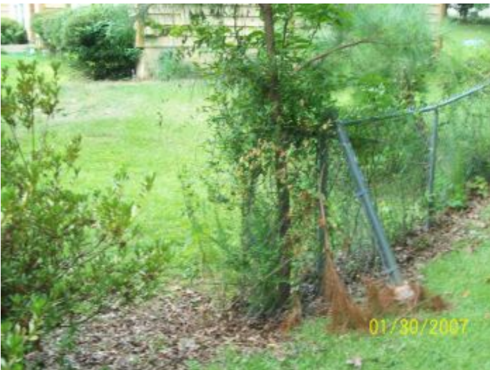
Gate and section of fence missing
