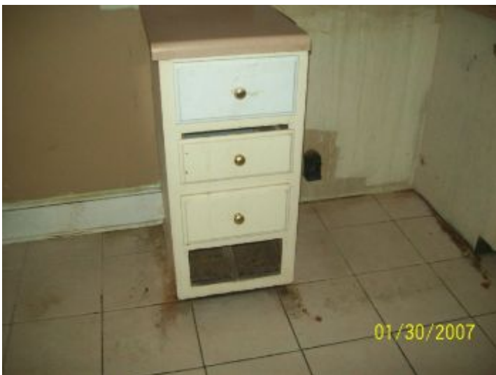
Drawer is missing
