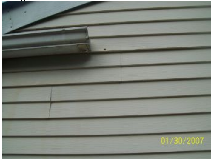
Downspout missing
